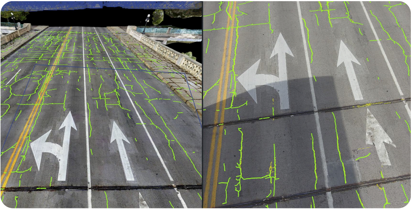
Analyze photos and get features for defect detection – Image courtesy of Collins Engineers
